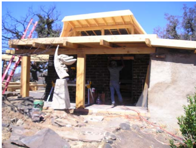
Mark Tighe and Office Construction
